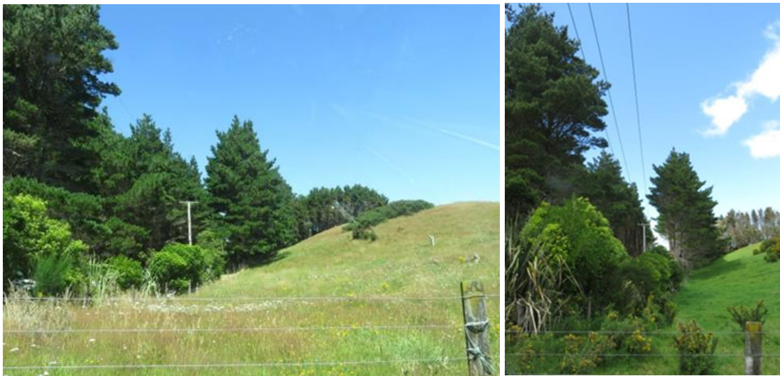
Figure 6-15 Covered Conductor Trial Installation Before (left) and After (right)
