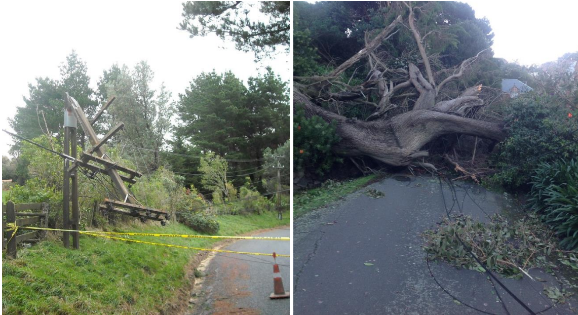
Figure 11-1 Storm Damage - June 2013
