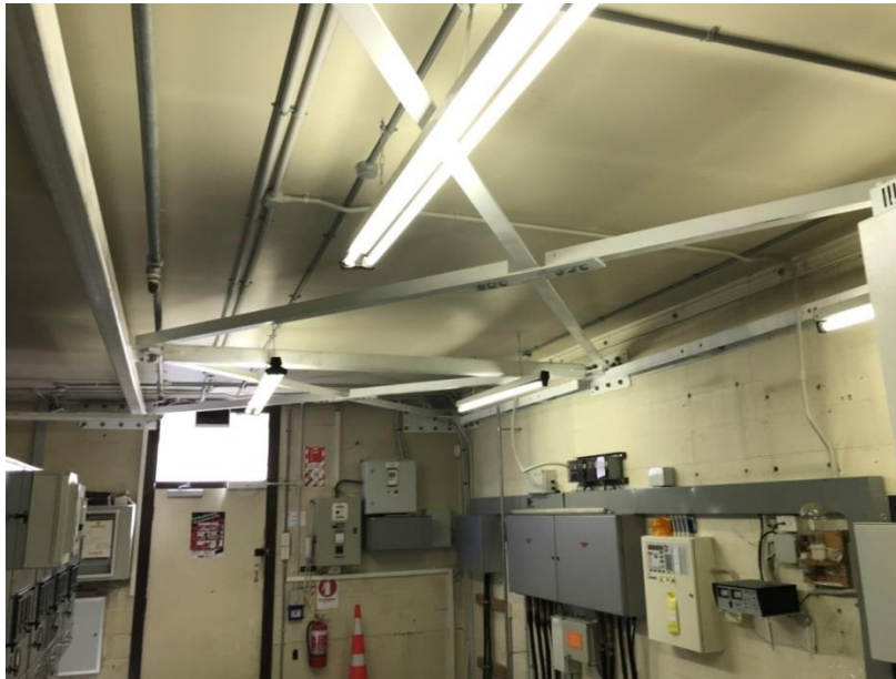
Figure 11-9 Seismic Bracing Installed inside Frederick St Zone Substation
