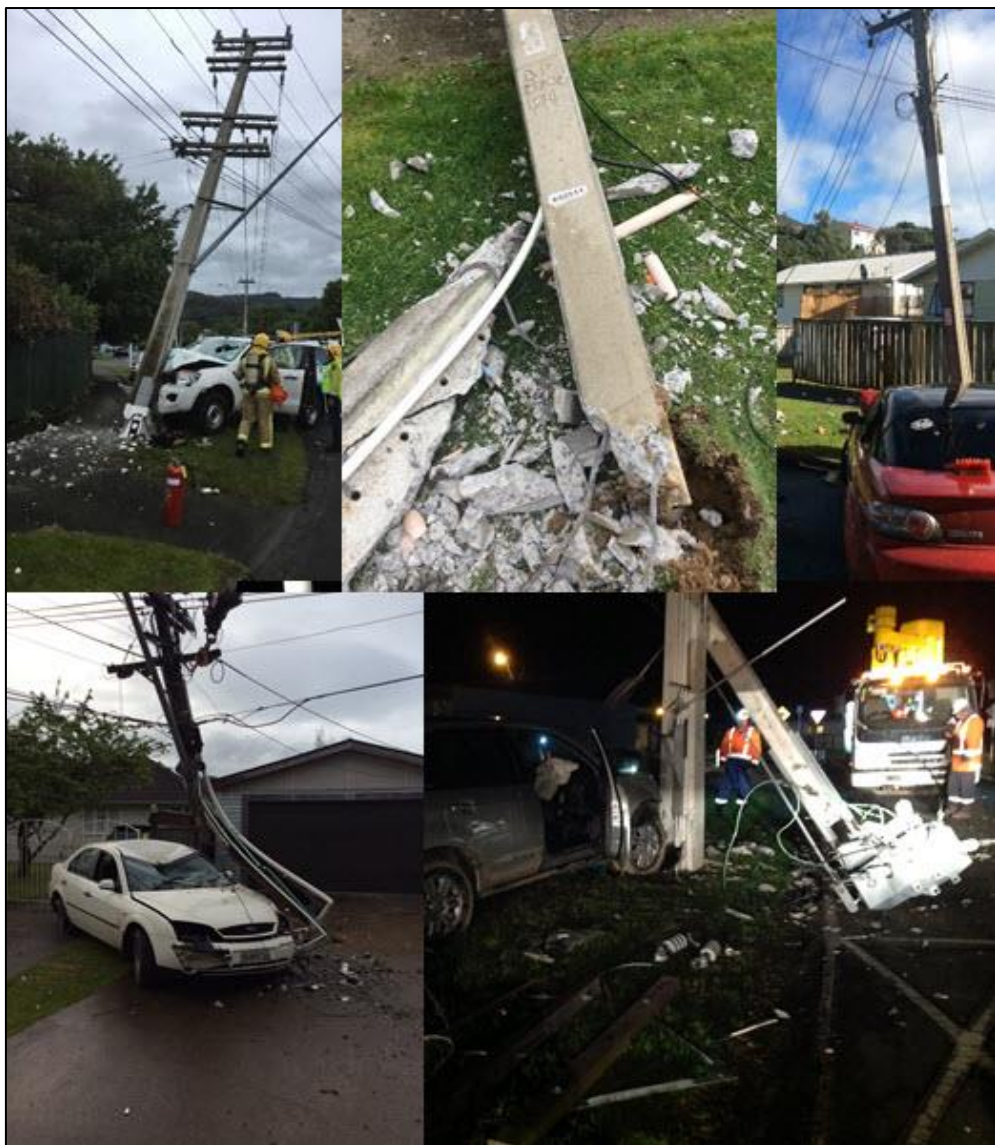
Figure 6-21 Fault Cause – Car versus Pole
