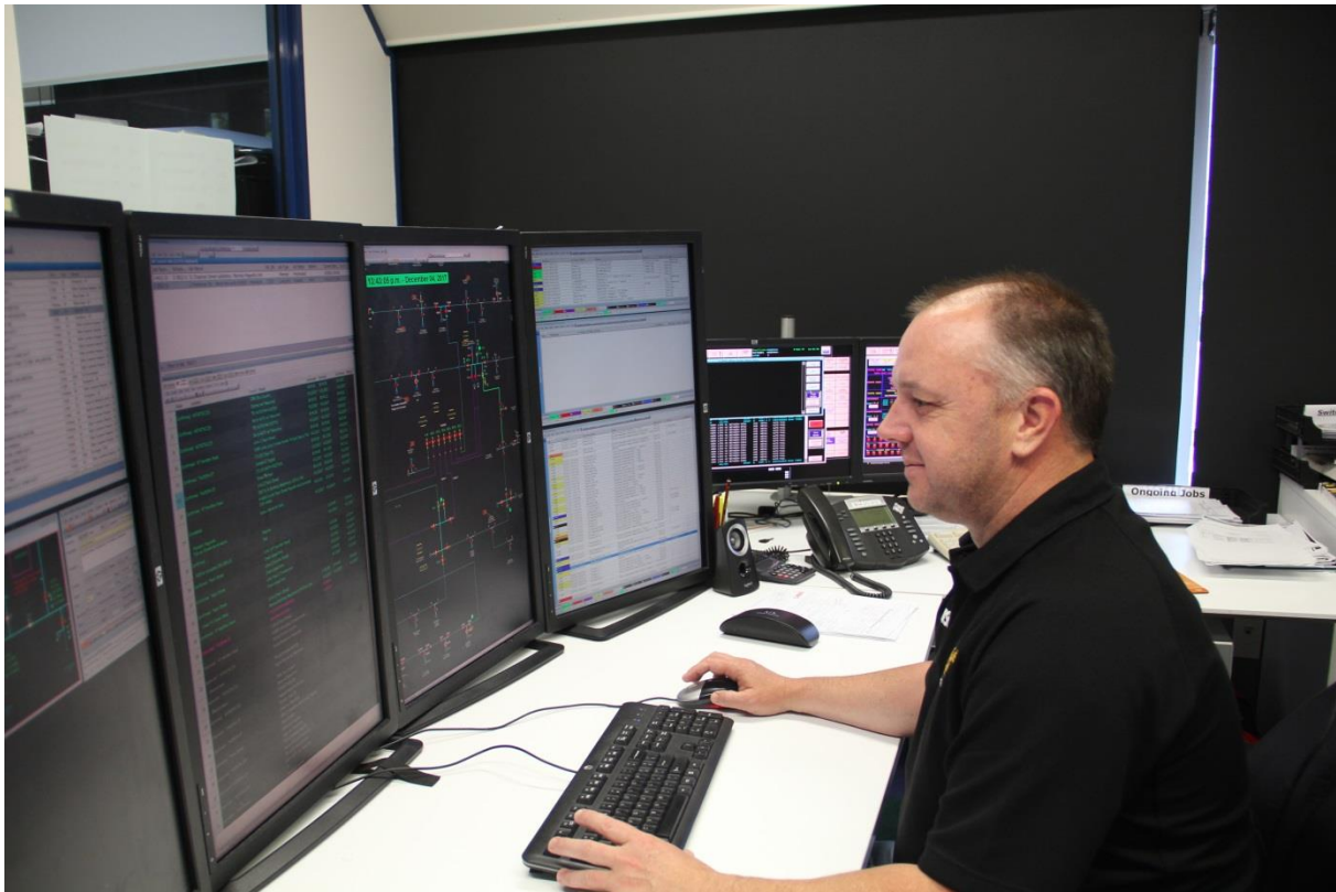
Figure 10-1 Main Network Control Room
