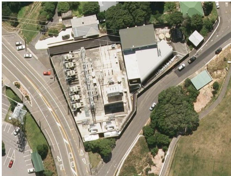
Figure 11-3 Central Park Substation
