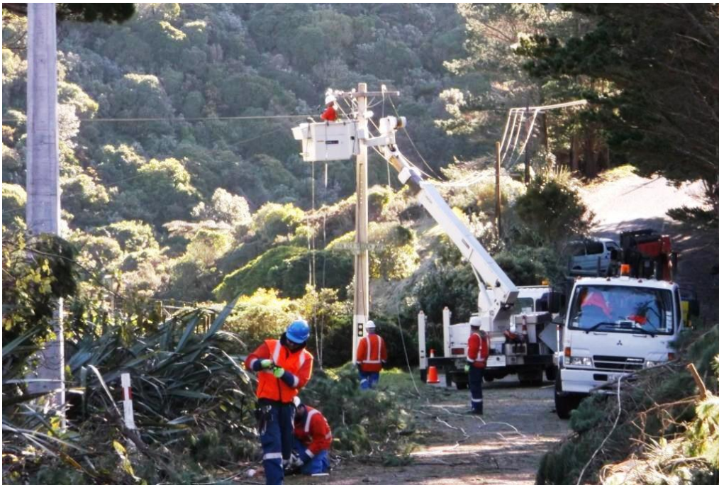
Figure 11-2 Contractors Working to Repair Storm Damaged Lines - June 2013
