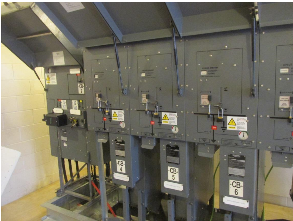
Figure 7-24 11kV Switchgear Replacement at 541 Hebden Crescent Substation
