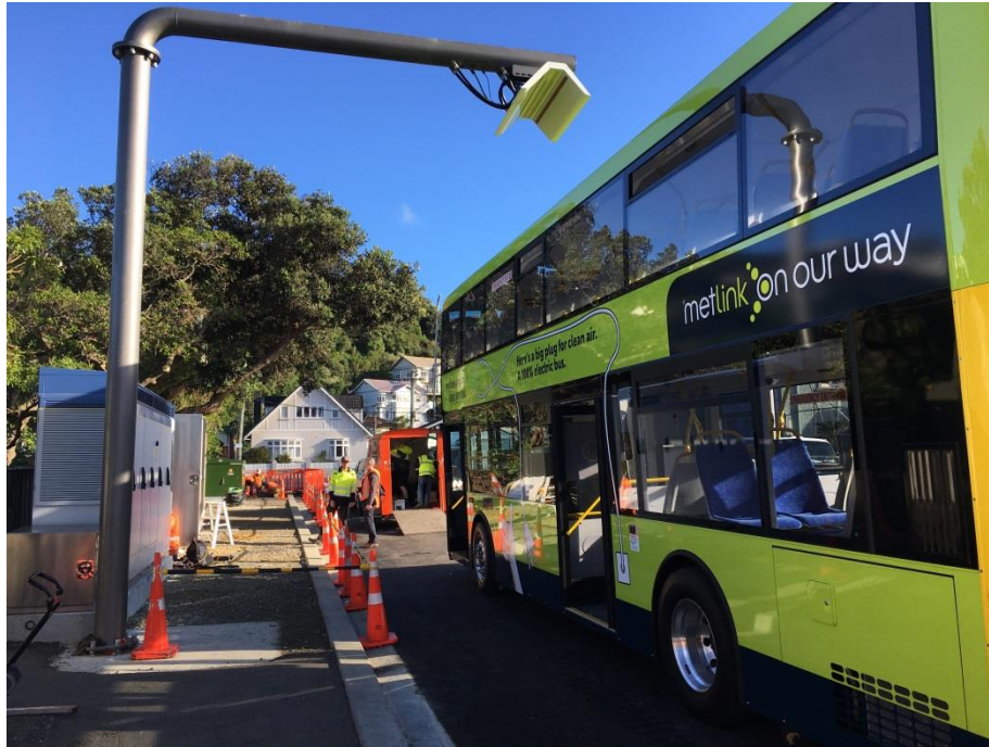
Figure 9-11 Electric Bus using a Pantograph Fast Opportunity Charger on WELL network
