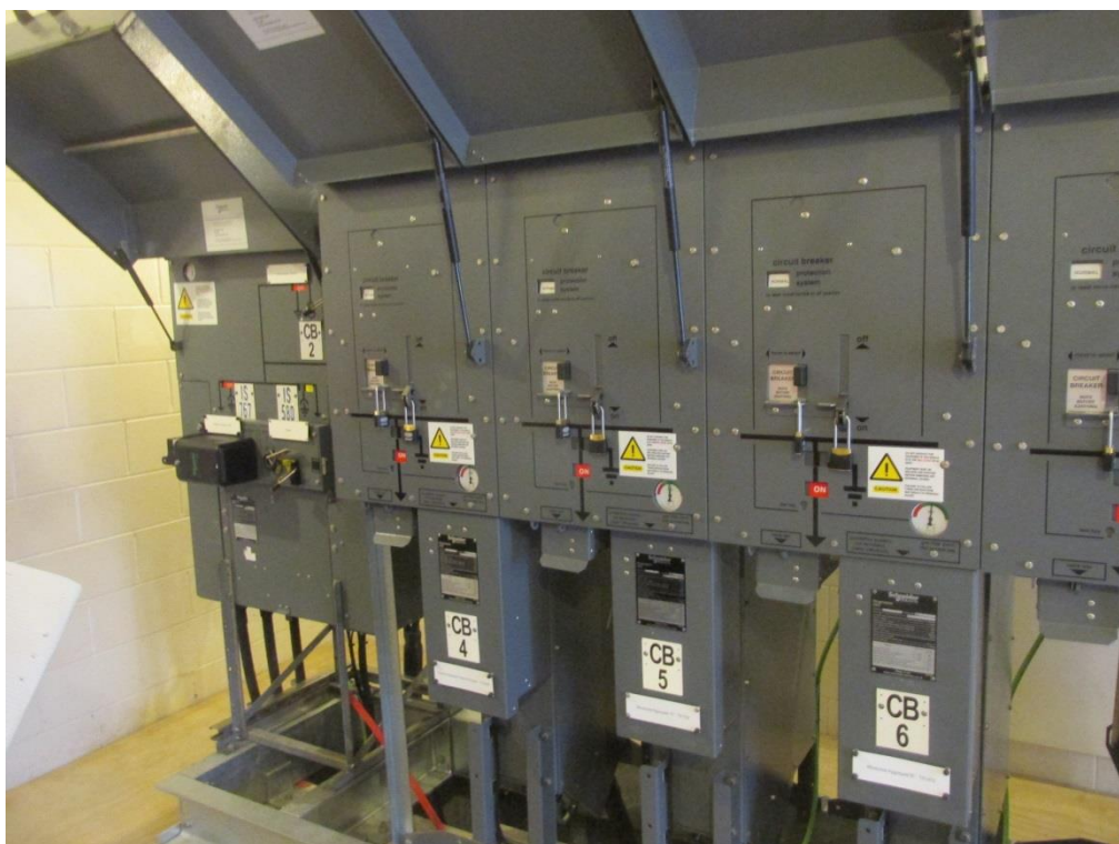
11kV Switchgear Replacement at 541 Hebden Crescent Substation
