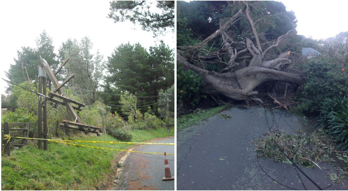
Storm Damage - June 2013
