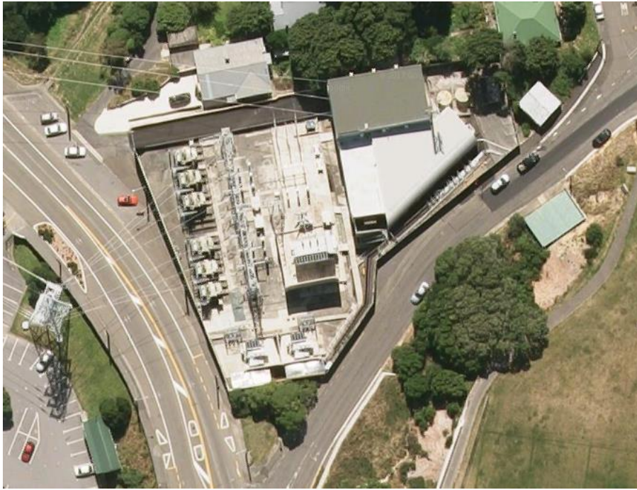
Central Park Substation
