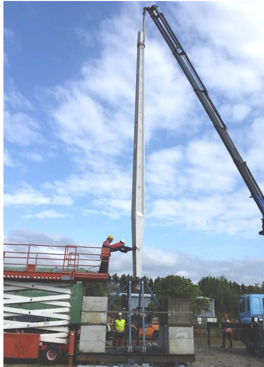
Large Foundation Being Prepared for Testing
