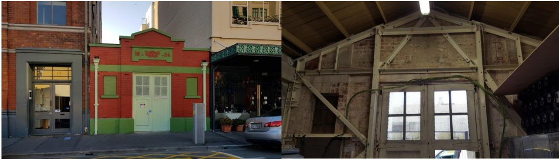
Exterior (L) and Interior (R) of Tory Street Substation
