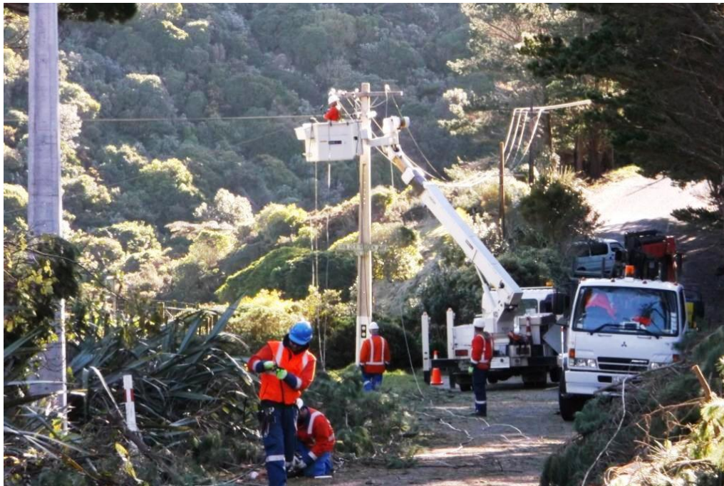
Contractors Working to Repair Storm Damaged Lines - June 2013
