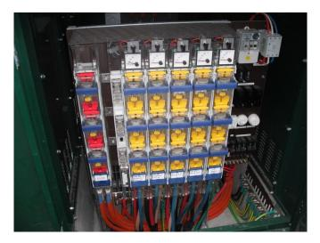
Photo of Low Voltage Disconnect Switches/Fuses
