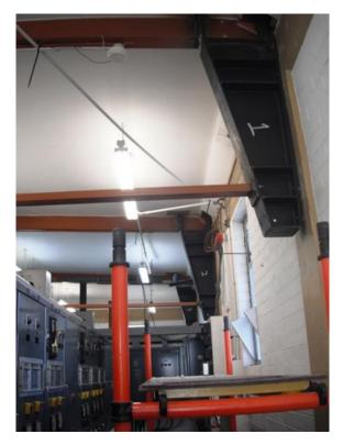
Figure 5-14 Seismic Strengthening at Gracefield zone substation
