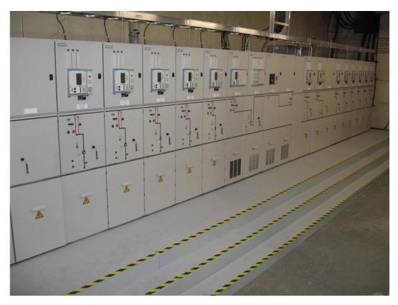
Photo of an 11 kV Circuit Breakers at The Terrace Zone Substation
